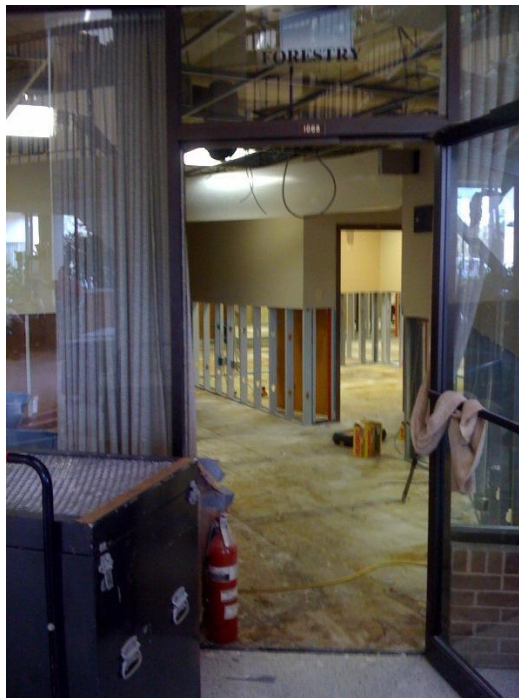
Figure 27: Office of Forestry after Hurricane Gustav
