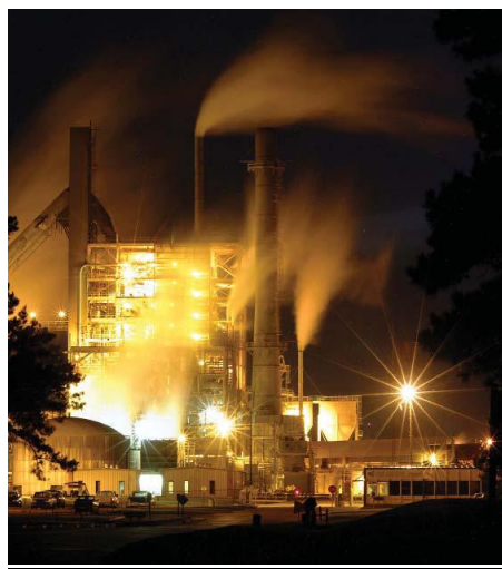
Figure 5: Like most pulp/paper mills, International Paper Company's mill near Pineville, La., burns bark and wood waste in its boilers to generate both heat and electrical power.
